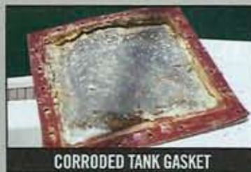
CORROSION, PITTING & RESIDUE
